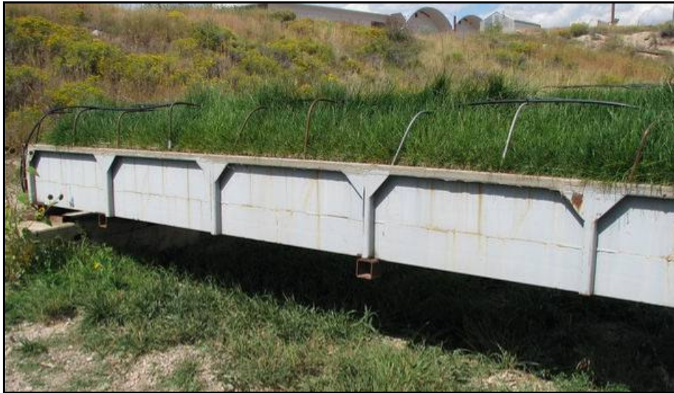
Figure 1-1: Photograph of ScourStop TM with Kentucky Bluegrass
