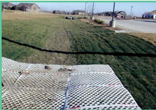
Flow transition mats installed below large culvert outlet.
